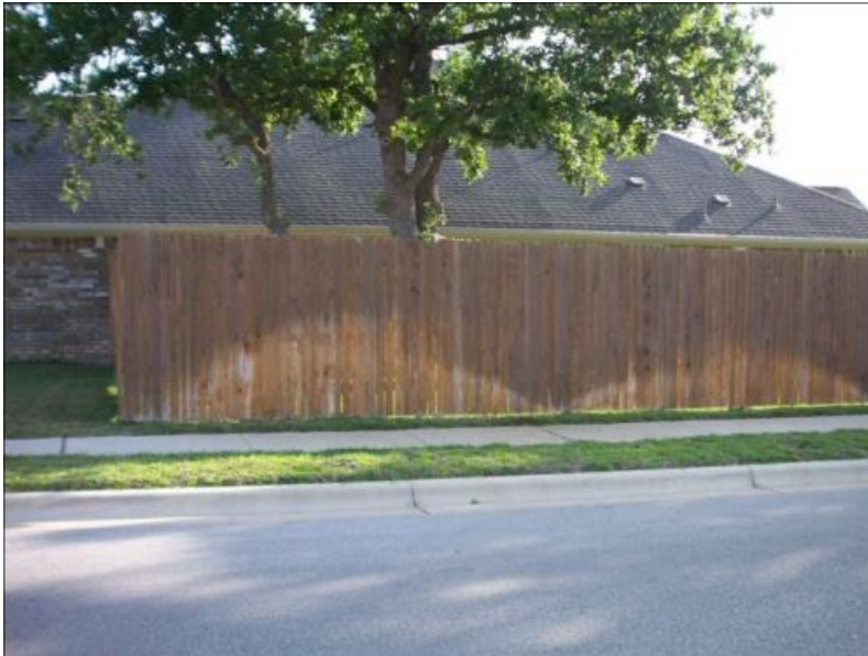
Example 1: Sprinkler Pattern has completely removed stain from bottom half of pickets.
